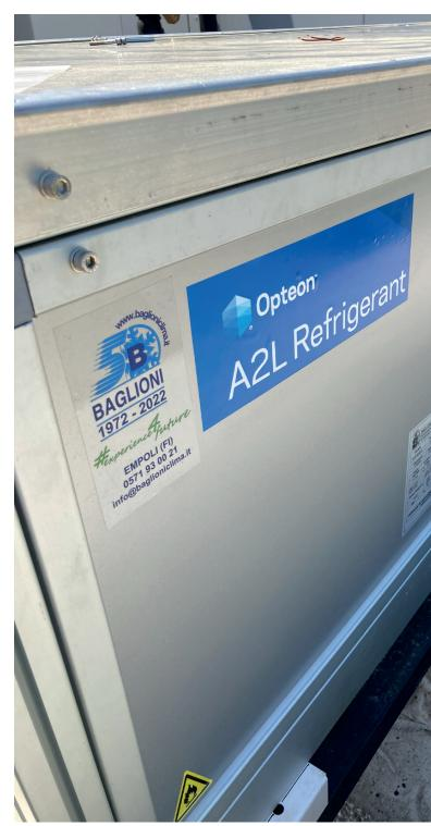
Opteon<sup>™</sup> XL20 (R-454C) has proven to be an excellent replacement for R-404A, suitable for ensuring the high performance required for the operation of production processes, while reducing direct emissions into the environment by 96%.
